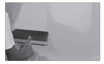
Compound buildup on the active surface of the speaker should not exceed 3mm (1/8").
