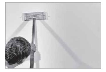
16. Validate the finish thickness using the Sonance DISC system and DG-1 depth gauge (SKU 93491).
