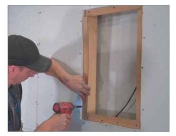
9. Connect the speaker wire from your wall or ceiling to the terminals on the speaker.
